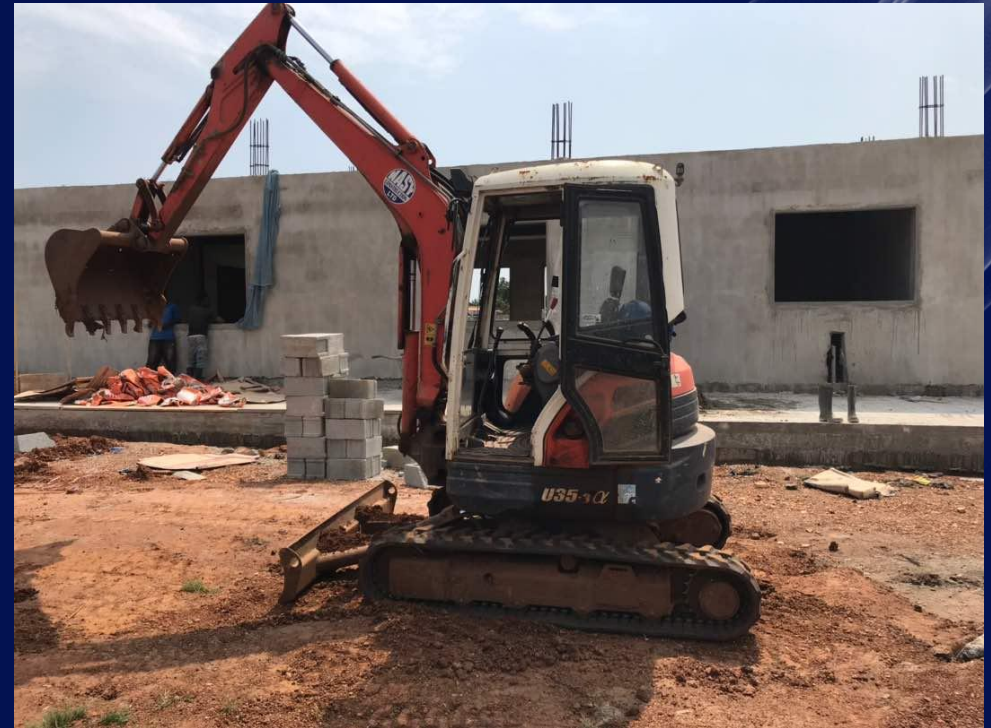
KUBOTA 3TON EXCAVATOR
